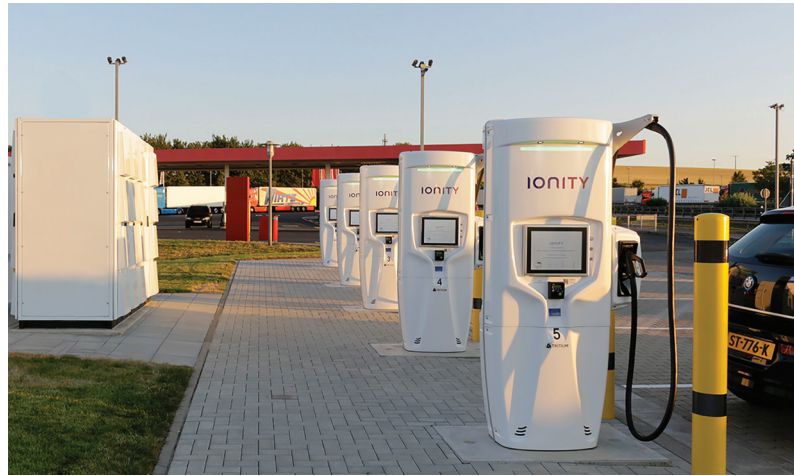
PK system, Brohltal-Ost, Germany. Image used with permission of IONITY.
