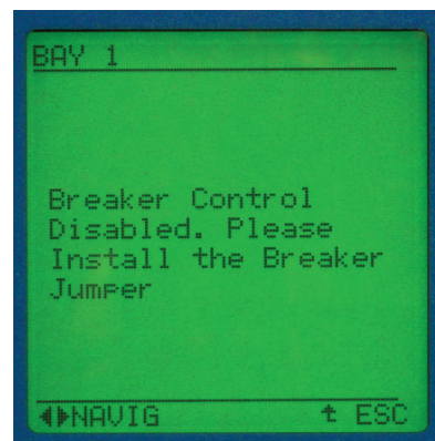
Breaker Control Disabled Message (Figure 6c)
